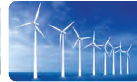
海洋风电塔筒 Offshore wind tower
