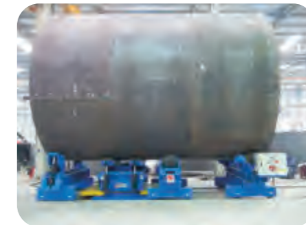
组对完成后由操作机焊接内外环缝 Welding inner & outer circular seam after finish fit up together
